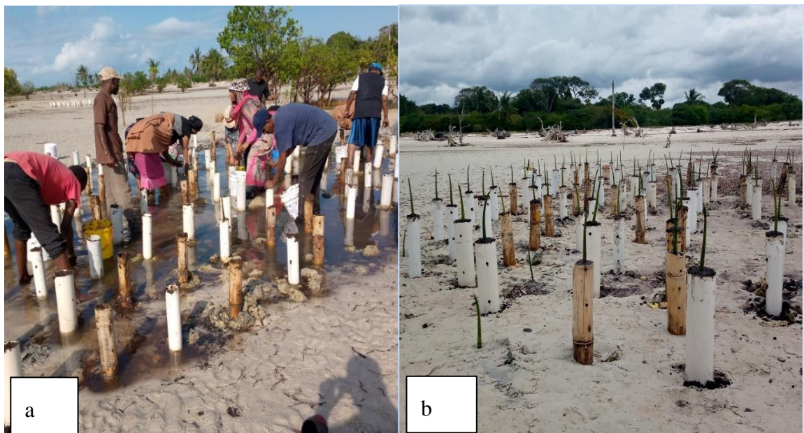
Figure 5: (a) Sediment filling within the installed encasements and (b) newly planted mangrove seedlings.
