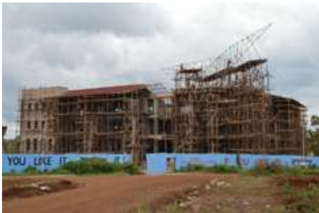
Modern Library Under Construction
