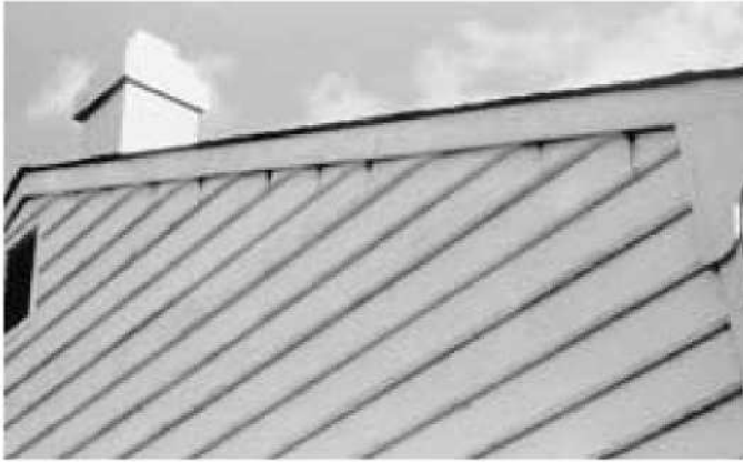
Figure 6.20. Carpenter bee damage.
