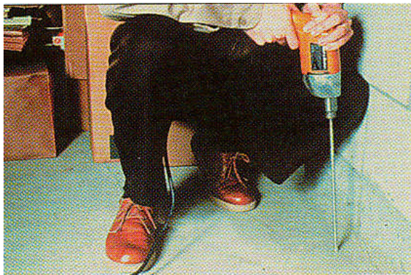
Figure 3.5. Slabs are drilled so that termiticide can be injected through holes to treat the soil beneath.
