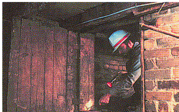
Figure 3.9. Inspection of crawl space for termite infestations (he should also be wearing gloves).
