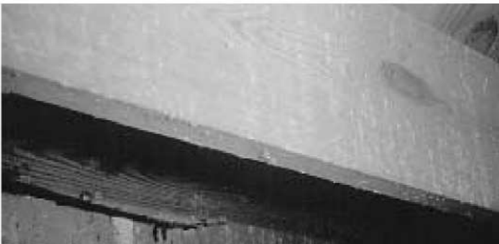
Figure 6.2. Anobiid beetle damage in pine floor joist—note frass being pushed out of old exit holes (USDA Forest Service).
