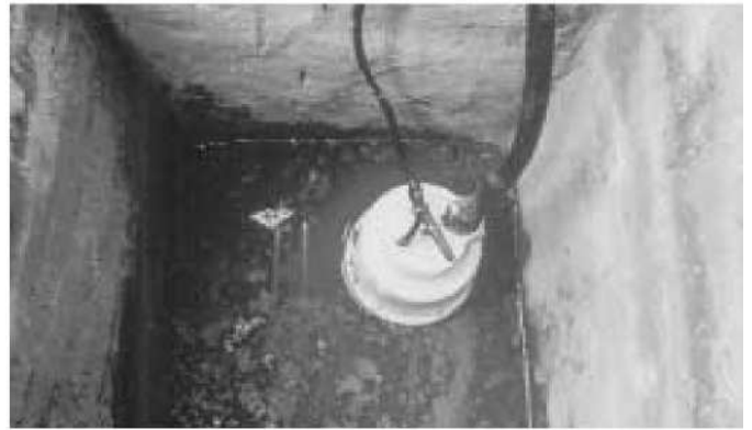
Figure 5.5. If the basement has a sump pump, care should be taken to avoid getting chemical into the “sump” or pit in which the pump sits. This is important because sump pumps usually discharge into non-target areas, such as a driveway, street gutter, or underground sewer.
