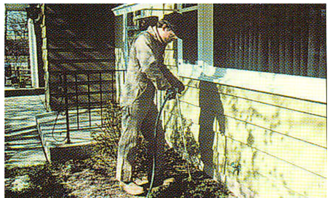
Figure 3.3. Pest management professional applying termiticide to the soil by long rodding the exterior of a house.
