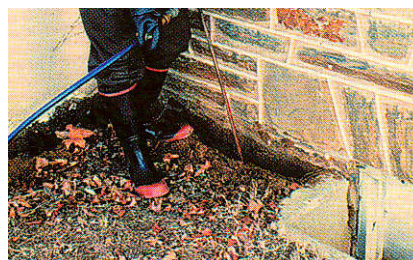
Figure 4.7. A typical basement treatment will also include trenching and rodding the outside perimeter of the foundation.
