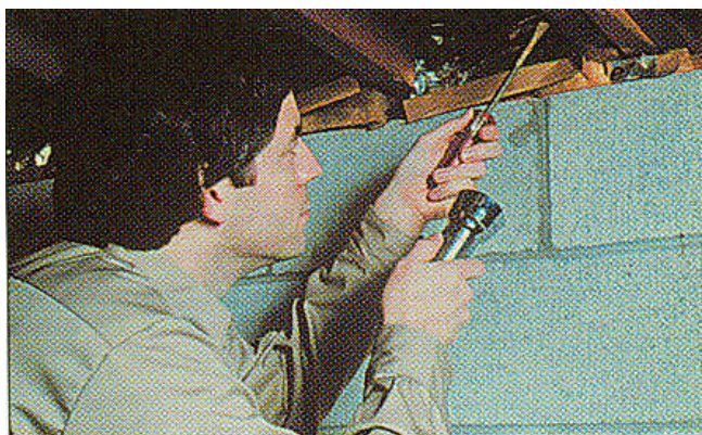
Figure 3.13. Probing the wood with a tool can help detect cavities.
